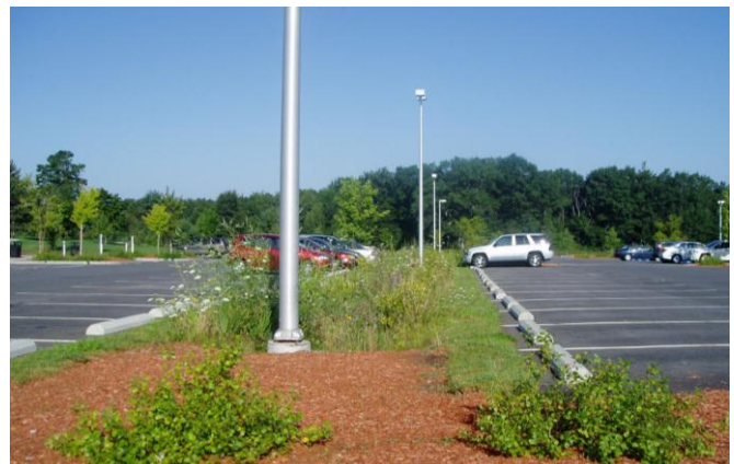
Low-Impact Development parking lot design (biofiltration)
