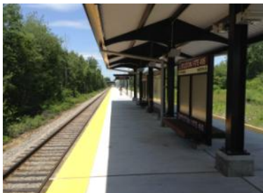
Littleton train station new raised platform for universal accessibility, safe and faster loading/unloading.
