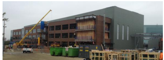
BMS new biologics development building, Dec. 2014
