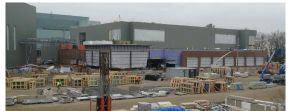
BMS new clinical manufacturing building, Dec. 2014
