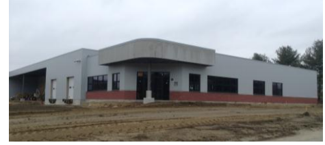
Maxant Industries new building shell – Barnum Road, Dec. 2014
