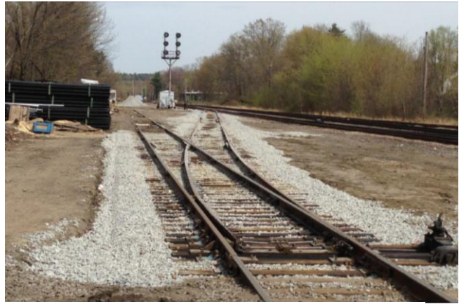
New cross-over track installed on Fitchburg Line in Ayer
