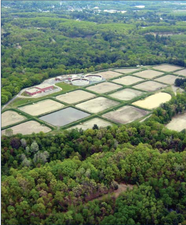
DEVENS WASTEWATER TREATMENT PLANT
