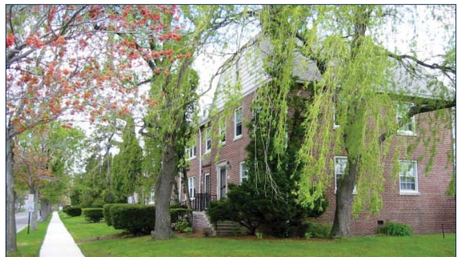
CHARACTERISTIC ROW HOUSES AT DEVENS
