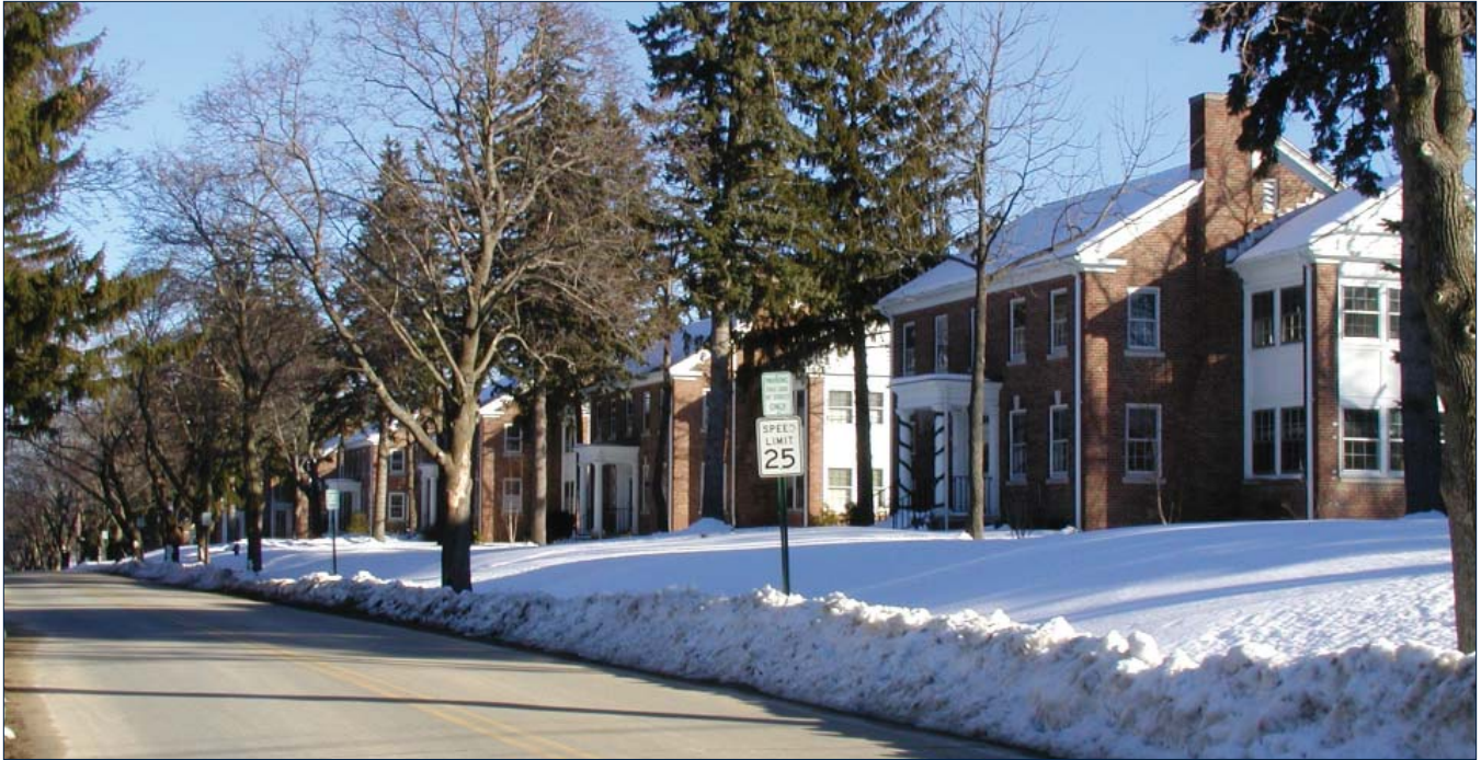
FORMER OFFICERS' HOUSING IN THE WALNUT AND ELM STREET NEIGHBORHOOD
