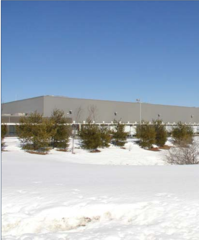
WAREHOUSE IN EAST RAIL INDUSTRIAL PARK
