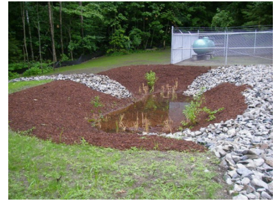
Bio-filtration basin at Patton Well. This system helps naturally treat and manage storm water runoff, protecting adjacent wetlands & promoting local groundwater recharge.
