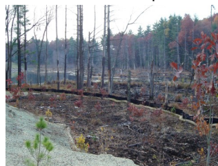
Created Wetlands—Patton Road. A stabilized slope leads into a created wetland area that blends into the existing wetland area.
