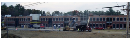
Systems H2O and Magna Motion—preparing for final Certificate of Occupancy—November 2008.
