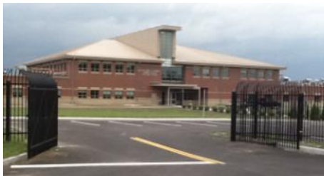
US Army —Training Building under construction on Barnum Rd.—July
