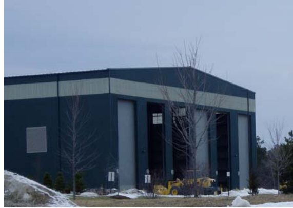
Three of six doors closed during routine inspection Dec 2009
