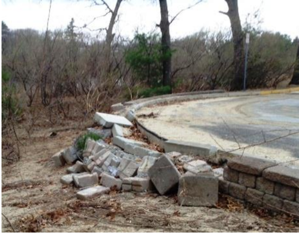
Retaining wall collapse – April 2014
