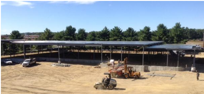
View of structural steel and roofing installation from the rear of the building
