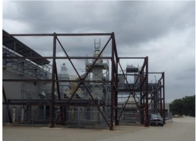
Sound wall and all noise generating equip. & duct work removed – Sept. 2014
