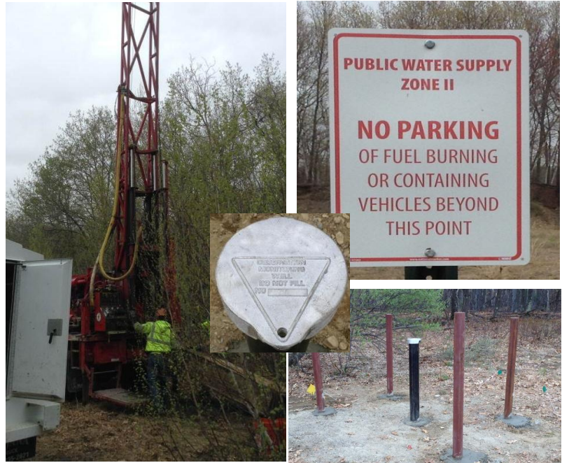
US Army groundwater monitoring well installation and signage May 2014.
