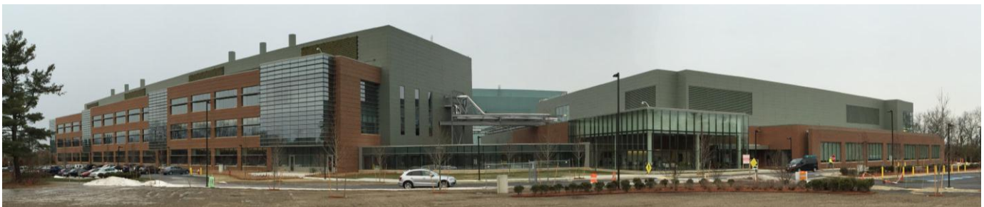
View of the front of the BDB (left) and the CMB (right) – January 2016
