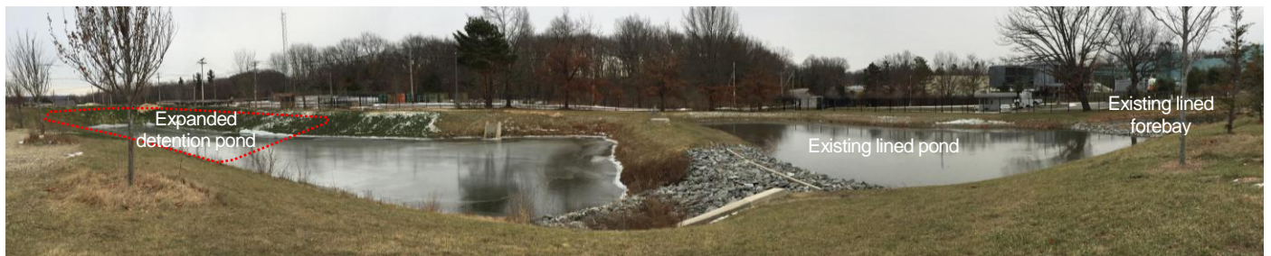
BMS newly expanded stormwater management basin in the rear of their facility (off of Queenstown Road). This system consists of a lined forebay and pond which treat stormwater runoff from the campus and can be isolated and contained in the event of a chemical spill. The third pond was expanded to accommodate a portion of the new development. It is unlined and provides groundwater recharge. January 2016
