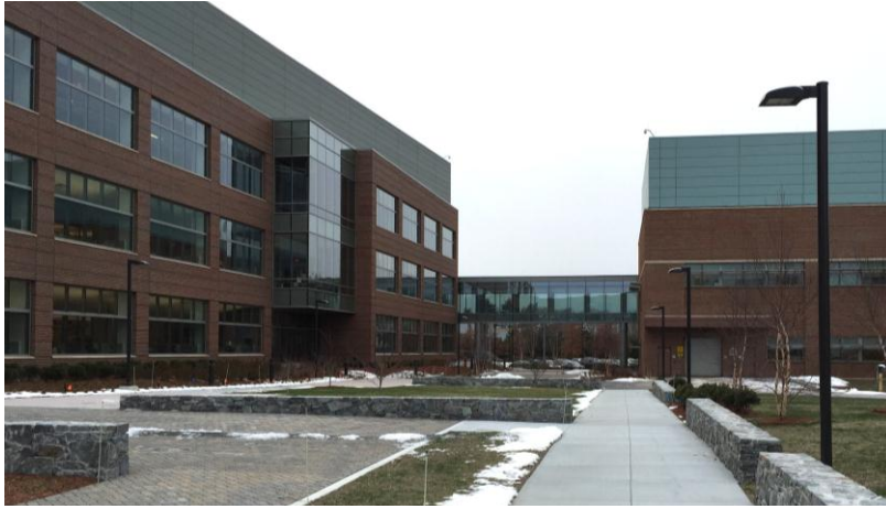
Rear of new BDB (left) and existing Lab-Office (right) connected by new elevated pedway. The courtyard underneath serves as a fire lane as well as an outdoor recreational/socializing space for employees. – January 2016
