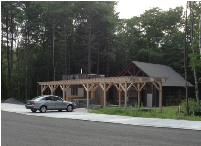
USFWS visitor contact station and parking. Pervious concrete parking area leading to composting toilets and the education pavilion. – July 2014
