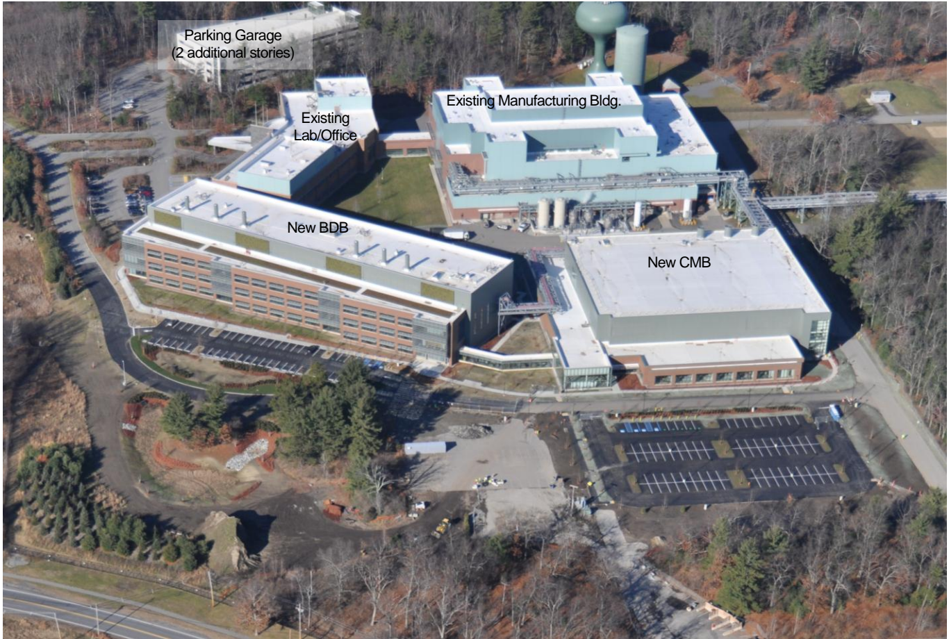
Aerial view of BMS upper Campus – December 2015
