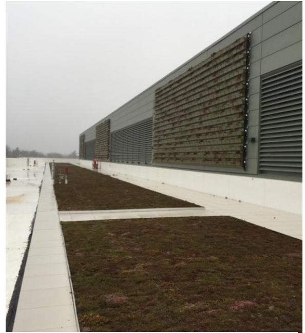
Green roof and green wall on the new BDB Building – December 2015
