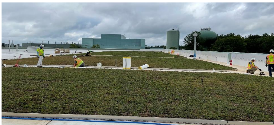
Vegetated roof installation on the CTF building- August 2021.
