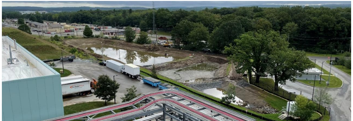
View of BMS stormwater management basins – lined forebay in the foreground, secondary lined treatment basin in the middle, and the third cell is the un-lined detention pond that allows for infiltration into the ground, with an emergency overflow structure drain into the Queenstown Road drainage system - August 2021
