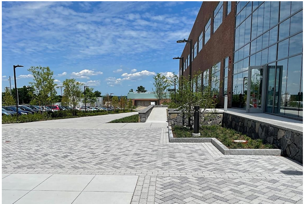
BMS's new Cell Therapy building pedestrian plaza and walkways featuring porous pavers – June 2022
