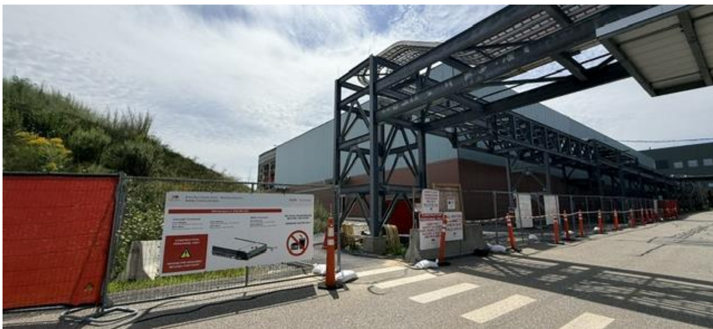
BMS Warehouse Expansion under construction – July 2026
