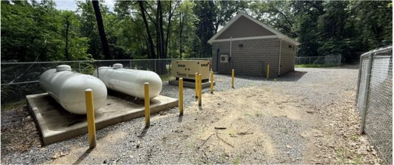
New booster pump station building and emergency generator and propane tanks for power back-up – July 2026
