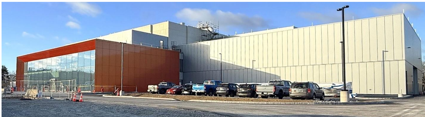
North end of CFS-2 Tokomak Hall – November 2025
