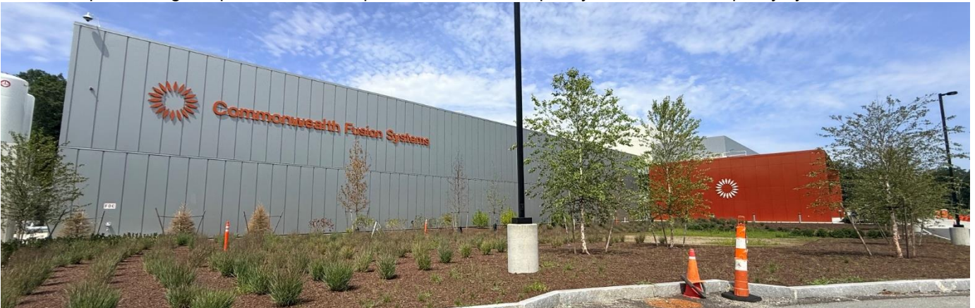
South end of CFS-2 Tokamak Hall – July 2026
