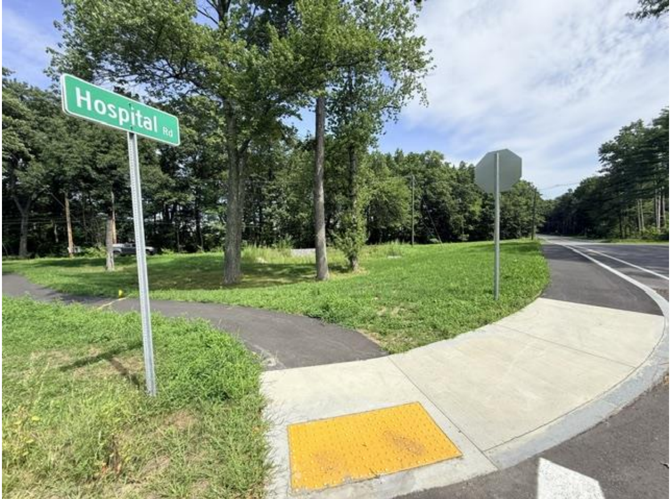
New sidewalks at the new intersection of Hospital Road and Givry Street. Mature tree preservation in the background and new low-impact development stormwater management features help decentralize and better treat and infiltrate runoff. – July 2026
