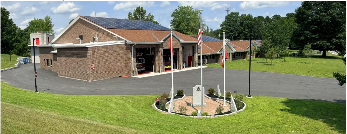
Rear of new Public Safety Building - Apparatus Bay, solar parking canopies, and fire training tower – July 2026.
