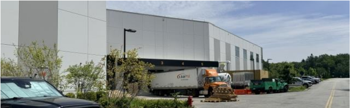
South side loading docks and utility yard of Vulcan Forms new location at 39 Jackson Road. August 2026
