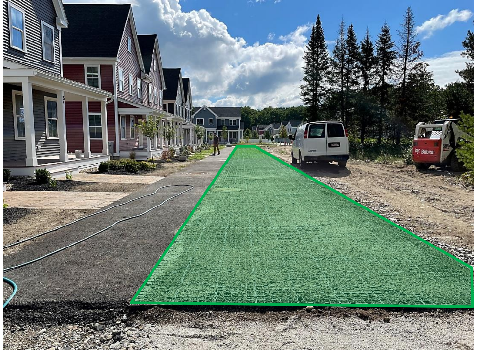
Powell Street duplexes fronting on Central Park. Green area is reinforced turf that will be all grass and blend in with the park when finished. Homes will be accessed via a public walkway through the park and via Powell Street (rear) – July 2022.
