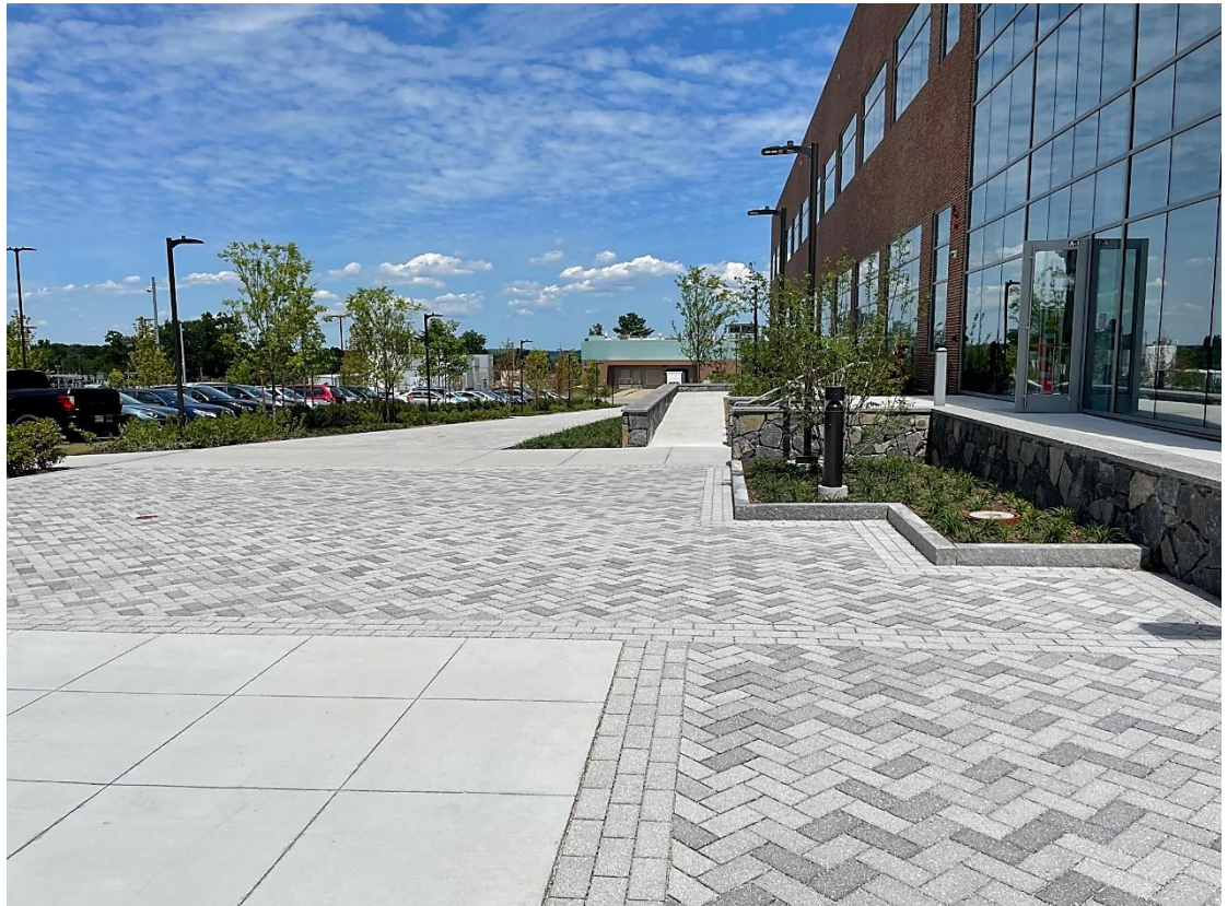
BMS's new Cell Therapy building pedestrian plaza and walkways featuring porous pavers – June 2022
