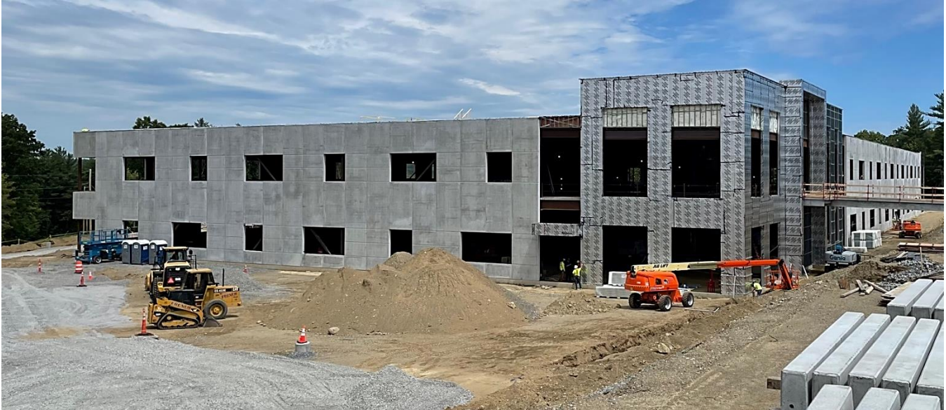
33 Jackson Road – rear building under construction – June 2022. Note the elevated walkway to the right which will be the main building entrance (2 nd floor), taking advantage of the sloping topography of the site. The first floor will be accessed via elevator, stairs or driveway.
