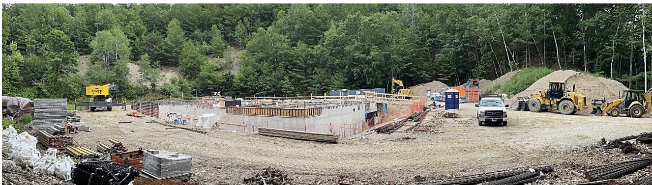
New Shabokin Water Treatment Facility off Sheridan Road: foundation walls and site work – June 2022
